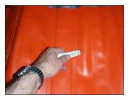
Damage to the base fabric must be repaired with a patch. To perform this type of repair, follow these steps:
