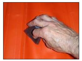
3. Wipe with a rag, dampened with solvent, to remove any residue from cleaning. Check to see if the area is totally clean and all coated surfaces and edges are dull. If not, repeat the cleaning. This is critical for a good glue bond.
