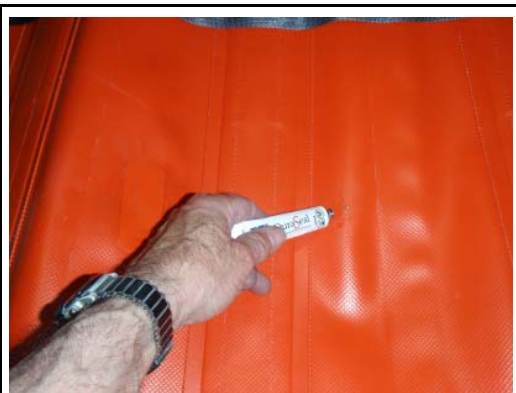
Squeeze glue around the tear and spread with fingers.
