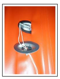
3. Pull the bolt up through the hole. Turn it until the clamp lines up with the hole.
