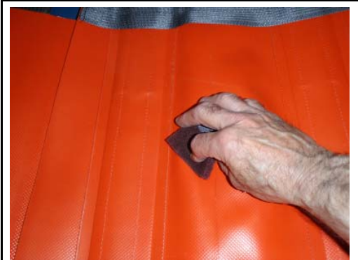
Clean and apply masking tape on the backside of the tear.
