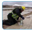
Personnel can now ready the tanks for filling by installing fill/drain valves to isolate individual tanks in the farm. Specialized arctic vents prevent overfilling.
