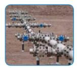
SEI Industries designed a customized fuel system that could face a number of challenges and in just three weeks, it was deployed and filled. The entire system was transported in 20-foot ISO containers. Here, the manifolds system is complete and is waiting to be connected to tanks.
