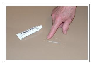
Place the patch and roll it down with the roller. Place the centre of the patch down first, then roll it out towards the edges.
