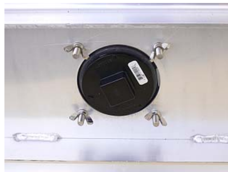
Flange installed in panel.
